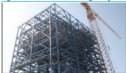
Figure 1: Boiler Structure Getting Ready
