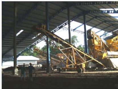
Figure 5: Crusher & Screening Plant
